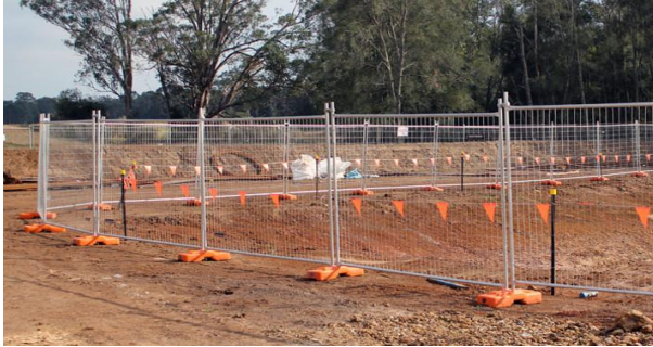
"Safety First #TemporaryFenceExcellenceTeam"
